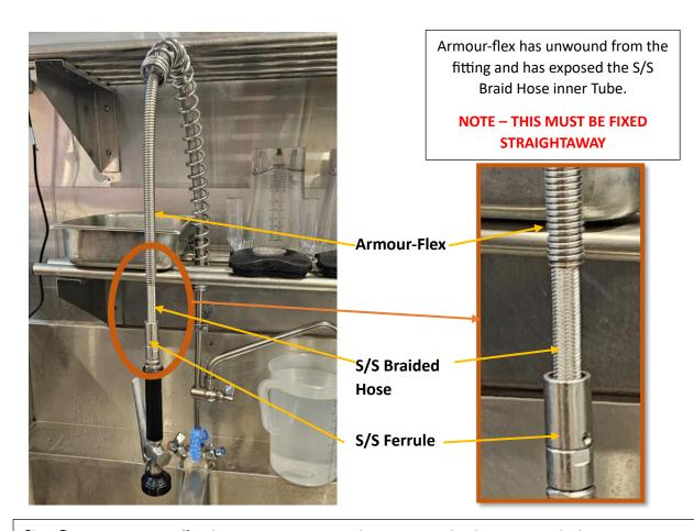
**<u>Step One</u>** - Turn Water Off and Squeeze Gun Trigger to let water out. This depressurizes the hose.
